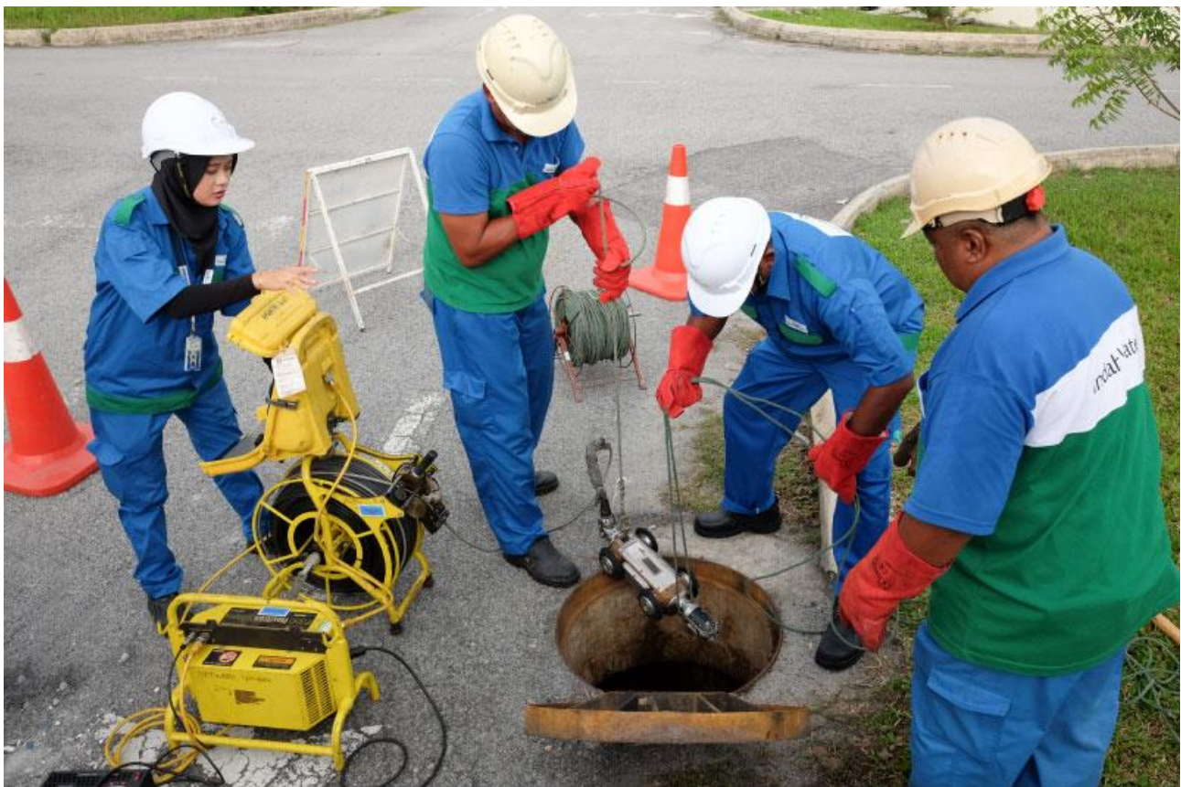
Figure 2 – Sewer CCTV inspection. Source: Indah Water Konsortium.
