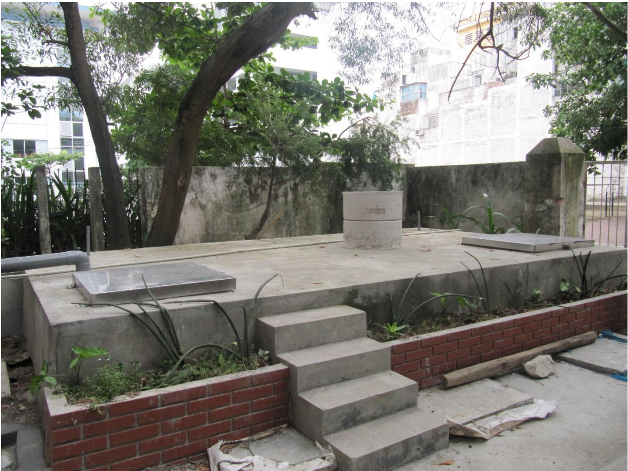
Figure 4 – Rainwater storage tank for flood mitigation in Hanoi University of Civil Engineering. Source: Hanoi University of Civil Engineering.
