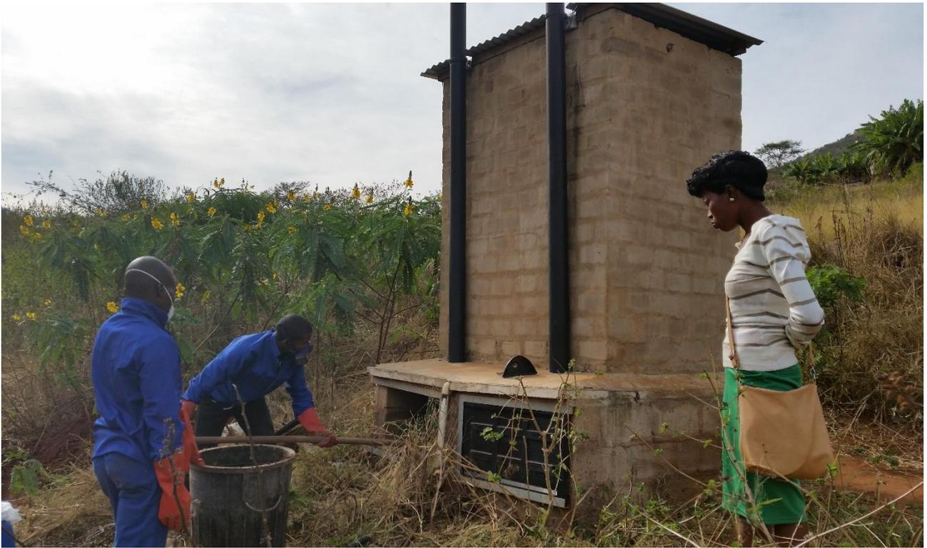
Figure 3 – Urine diversion dehydrating toilets (UDDT). Source: eThekweni Water and Sanitation.
