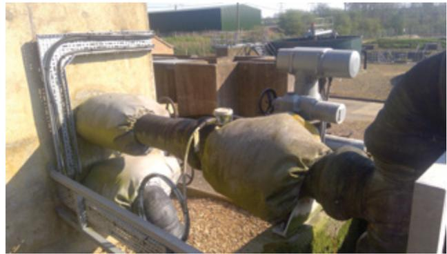
Figure 2.1 Poorly installed flow to full treatment flow meter
